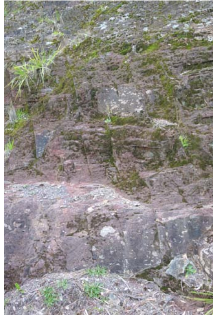
Figure 3.12: Joints in Bald Hill Claystone at Bald Hill
