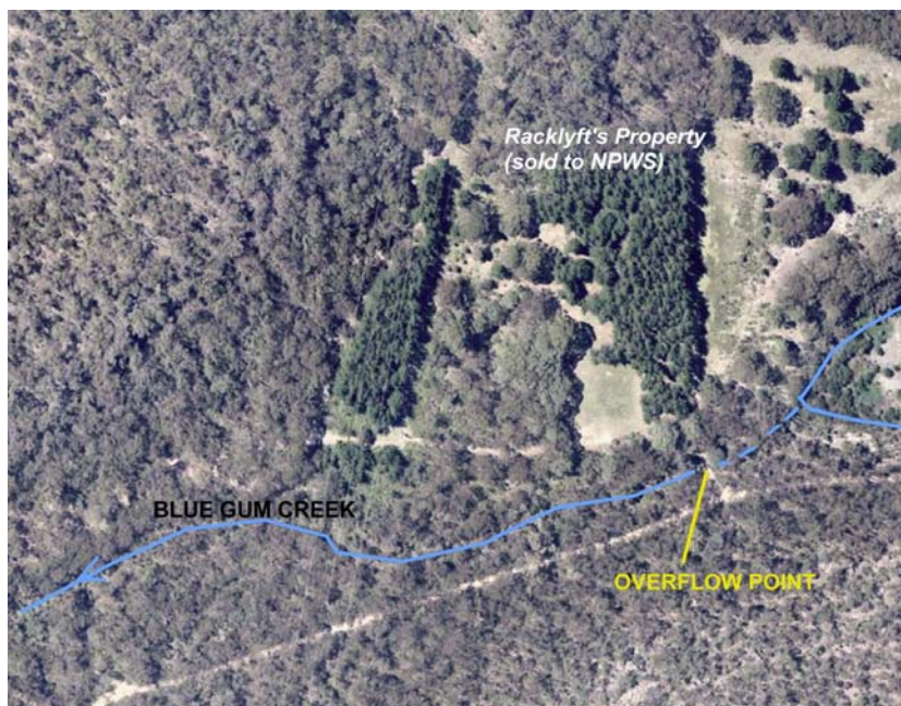
Figure 2.5: Overflow point between Lake Nerrigorang and Blue Gum Creek.
