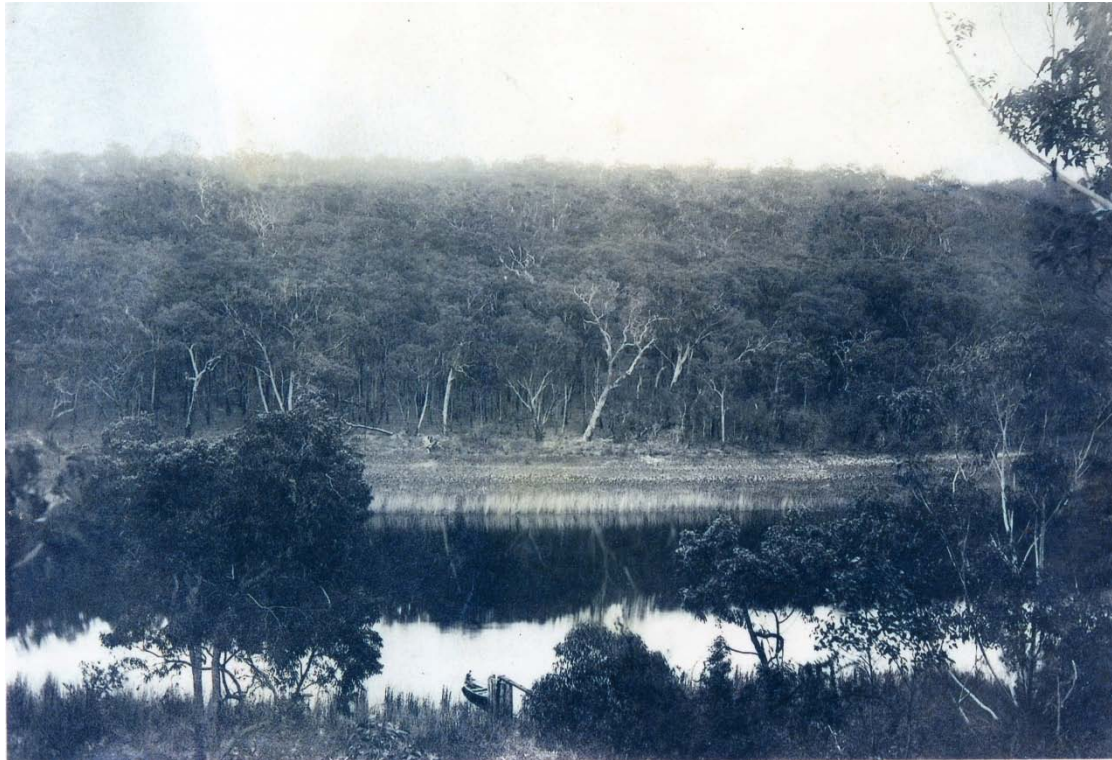
Figure 1: 1884 photograph of Lake Couridjah. Note inlet to Railways pump next to boat in lower centre of photograph.
